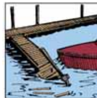
Property Damage to Docks
